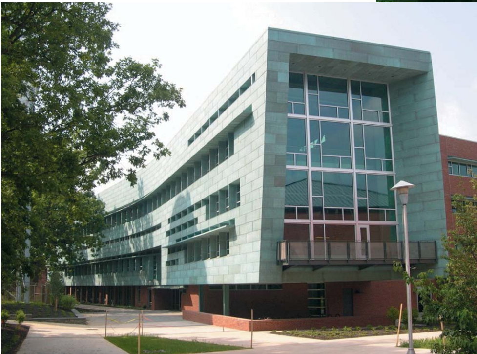
The copper cladding used traditional flat seam technique to tie the building into its more traditional surroundings.
