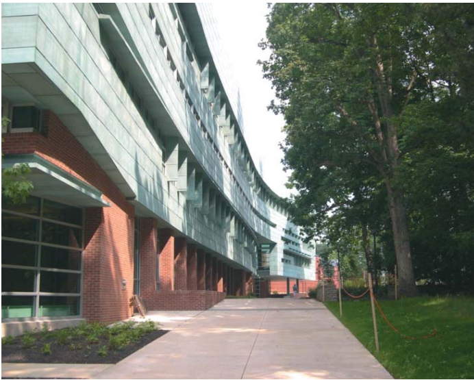
The pre-patinated copper clad South facing feature cradles and complements its existing surroundings. Photo: courtesy of Joe Nagy WTW Architects
