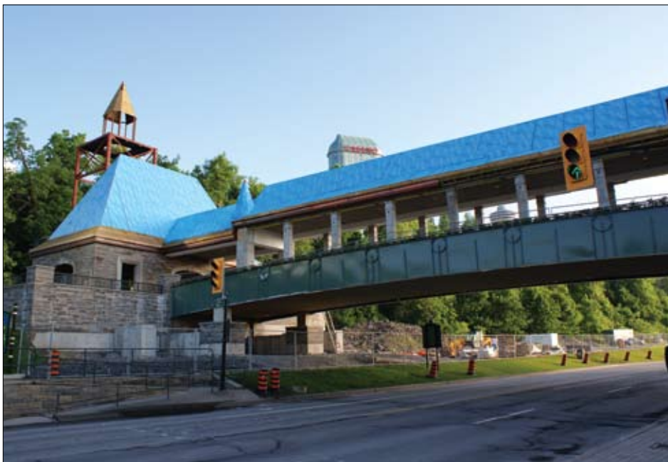
The new pedestrian bridge before installation of the copper.
