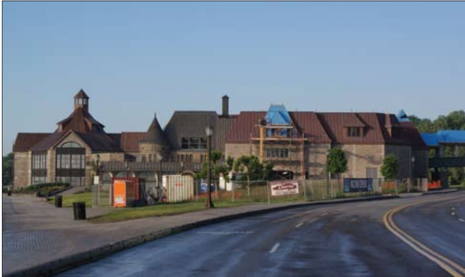
The project required over 70,000 pounds (31,000 kgs) of 20-oz copper sheet.
