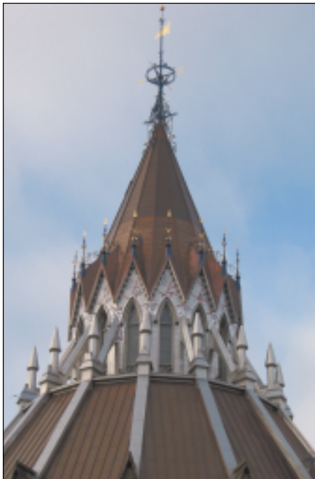
The lantern of the Parliamentary Library is topped with an ornate, refurbished spire.
