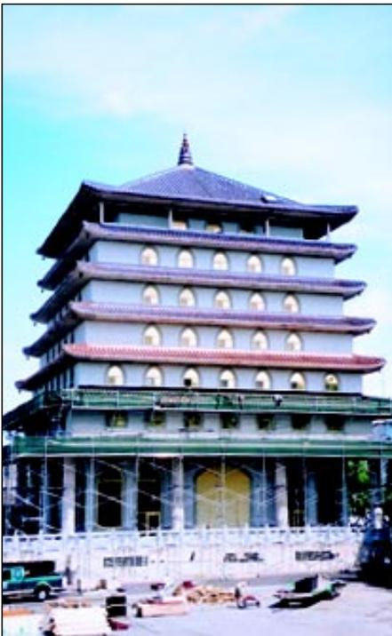
roof and first floor of the Temple. The total tonnage of the copper used for the Temple approaches 200,000 lb (90,000 kg).
