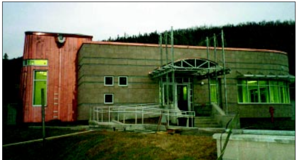
Copper is also used for the entrance canopy and flashings.
