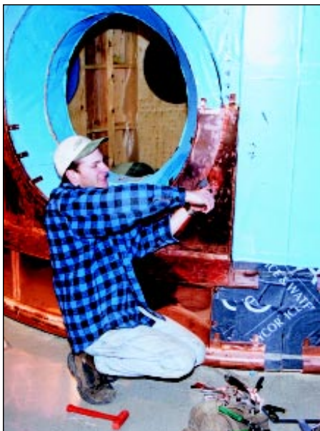
Cladding a window opening of the base of the dome.
