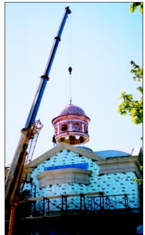
Hoisting the Holy Family Church dome.
