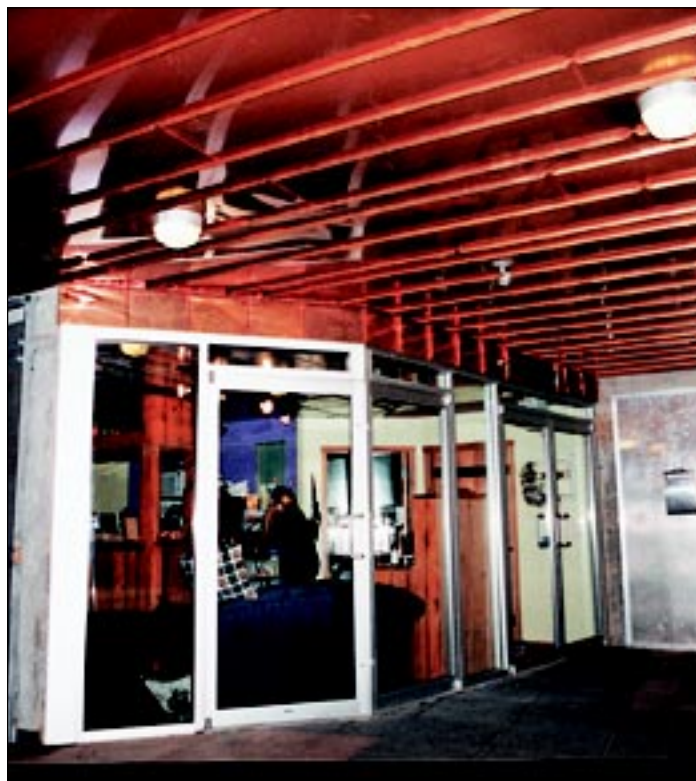
Copper was used throughout the project to add warmth and reflect light in areas that do not receive direct sunlight.
