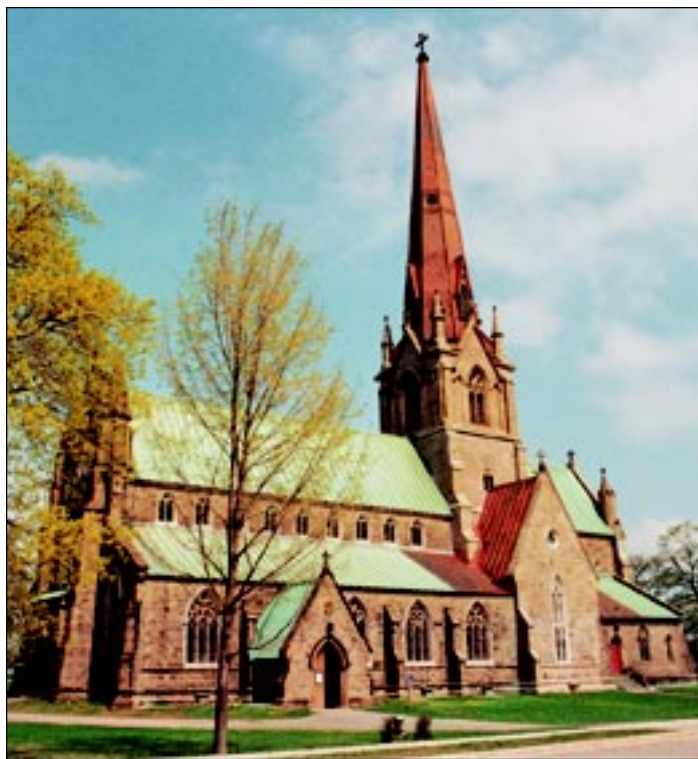
Christ Church Cathedral, showing the initial stage of the restoration.
