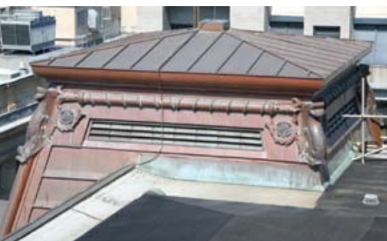
One of the four complex corner sections.
