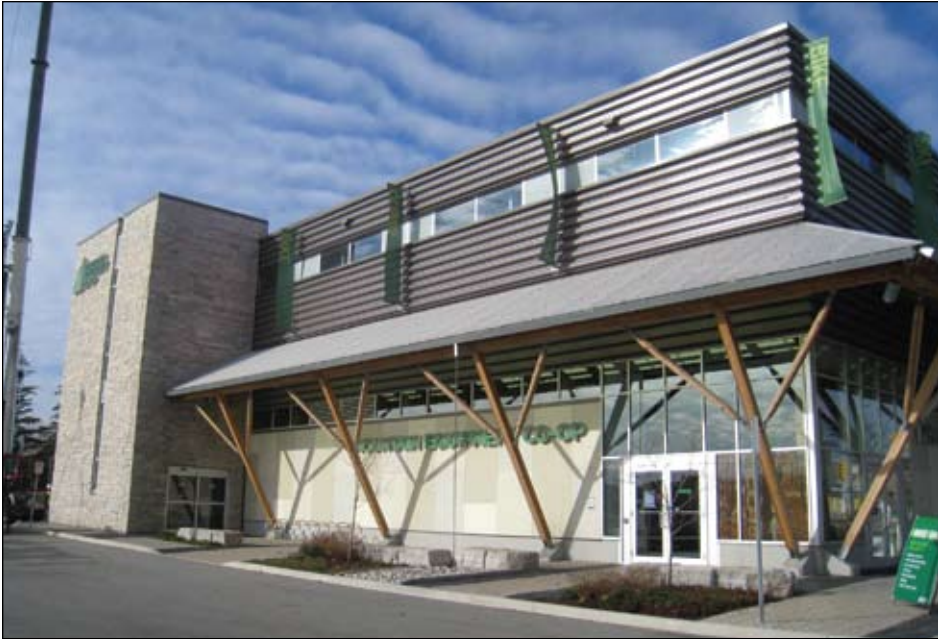
Mountain Equipment Co-op, Burlington, ON.
