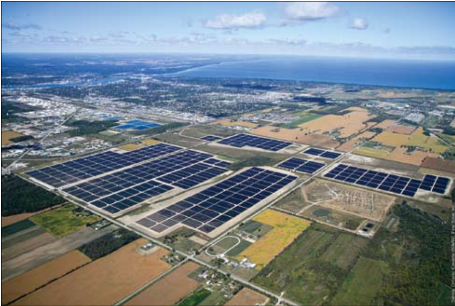
Aerial view of over 1.3 million photovoltaic panels covering about 650 acres (260 ha).
