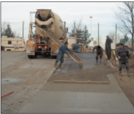
Pouring a concrete ramp during installation of electric radiant heating.
