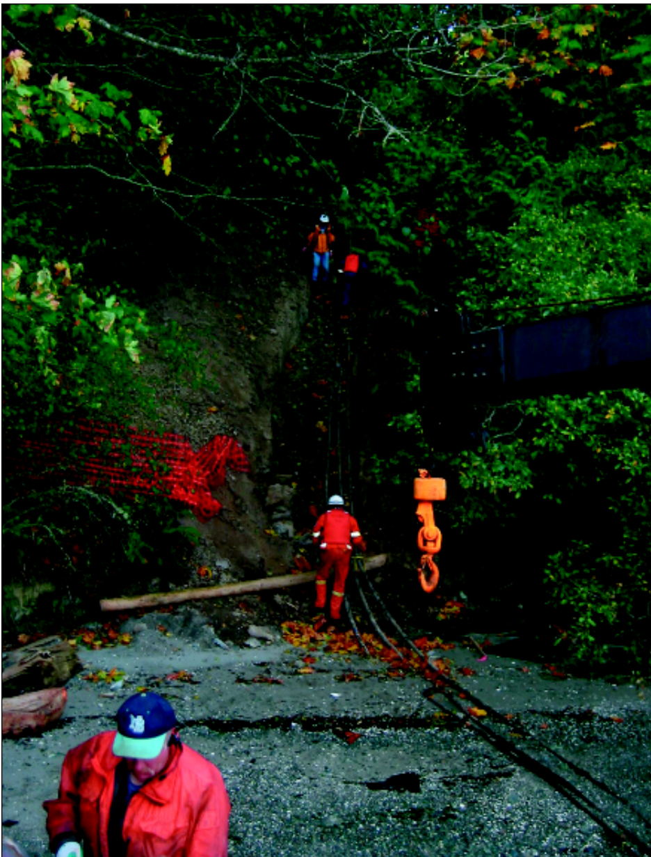
Removal of the existing 30-year old cable.
