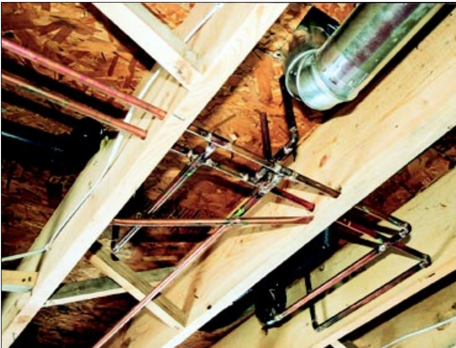
Compact hot and cold water supply lines fit in confined joist spaces.
