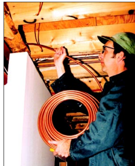
Lightweight copper tube is easily installed between joists.
