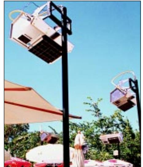
*Each infrared heater can heat an area of 110 to 160 sq. ft. (10-15m<sup>2</sup>).*
